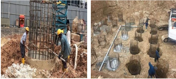
Gambar 4. Pondasi Bored Pile
